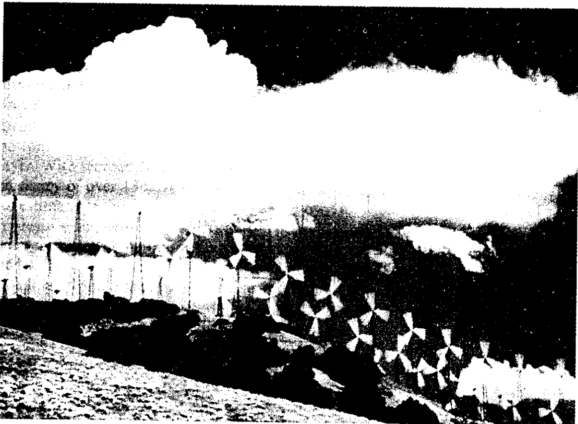
FIGURE 1.14. A wind-farm in Tehachapi Pass, CA with an overall installed capacity of 650 MW, enough electricity for more than 140,000 homes.
