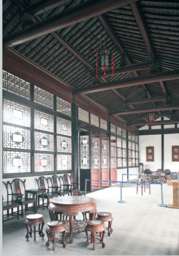
The wooden frame of a Chinese building (in this case part of the Suzhou Museum) 'where the walls are screens and not supports'.
