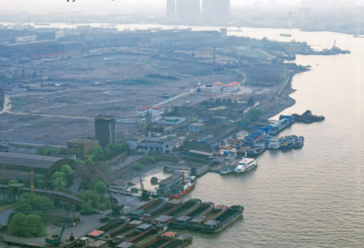
The Shanghai Expo site under construction on former shipyard land, 2007.
