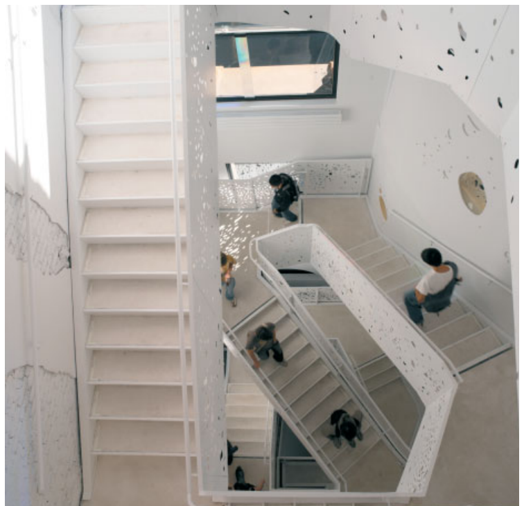
The larger perforated openings on the interior of the stair are made with USG Fiberock panels with Aqua-Tough (which allows them to be laser cut and submerged in water for extended periods of time). The Fiberock works seamlessly with the gypsum wallboard nearby, which is also painted white.
