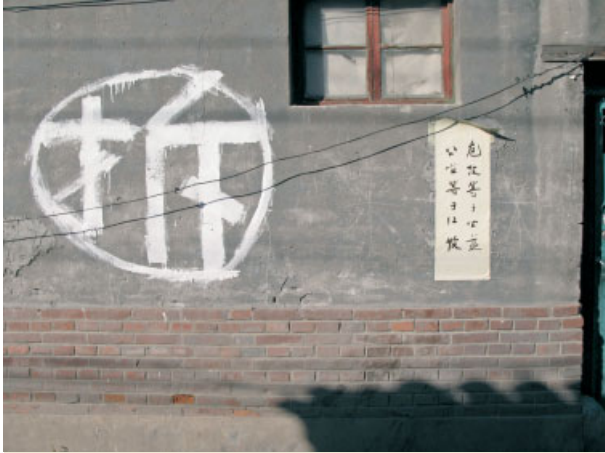
The Chinese character Chai (demolition) painted on the wall of an old house in Beijing in 2007 – a sign that the house will soon be torn down.
