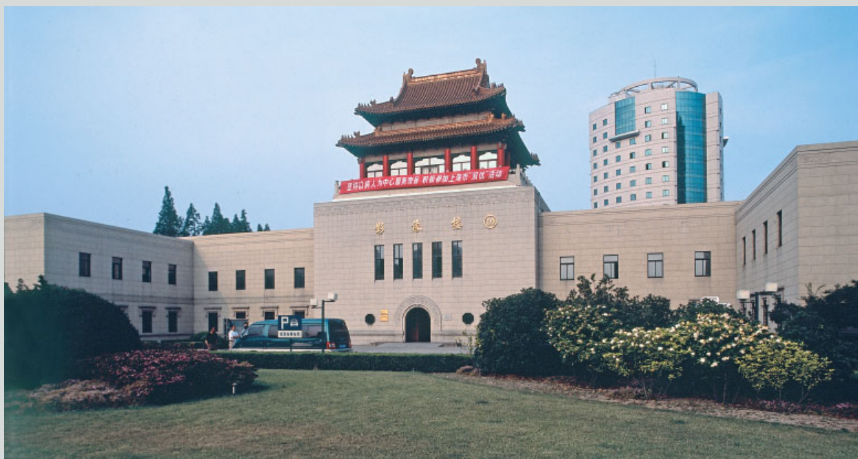
The former library in Shanghai's former Civic Centre, built in the mid-1930s, illustrating the often-criticised Chinese roof used to adorn modern structures to give them local 'meaning'.
