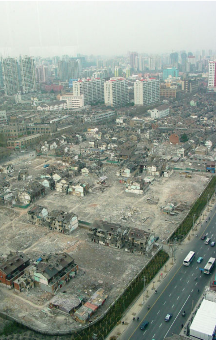
An inner-city construction site within the demolished old city fabric, Shanghai.
