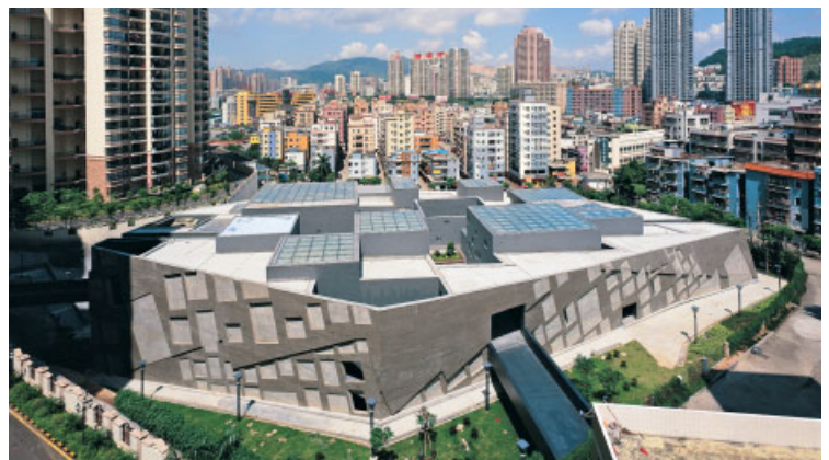
Dafen Art Museum, Shenzhen, Guangdong Province, 2007 The museum is a unique project for both the city of Shenzhen and for the museum's architects. Located on the outskirts of the city, in Dafen Oil Painting Village, which is best known for producing forgeries of world-famous (and obscure) paintings, this mixed-use art centre responds to both the topography and unique cultural setting of its urban environment.
