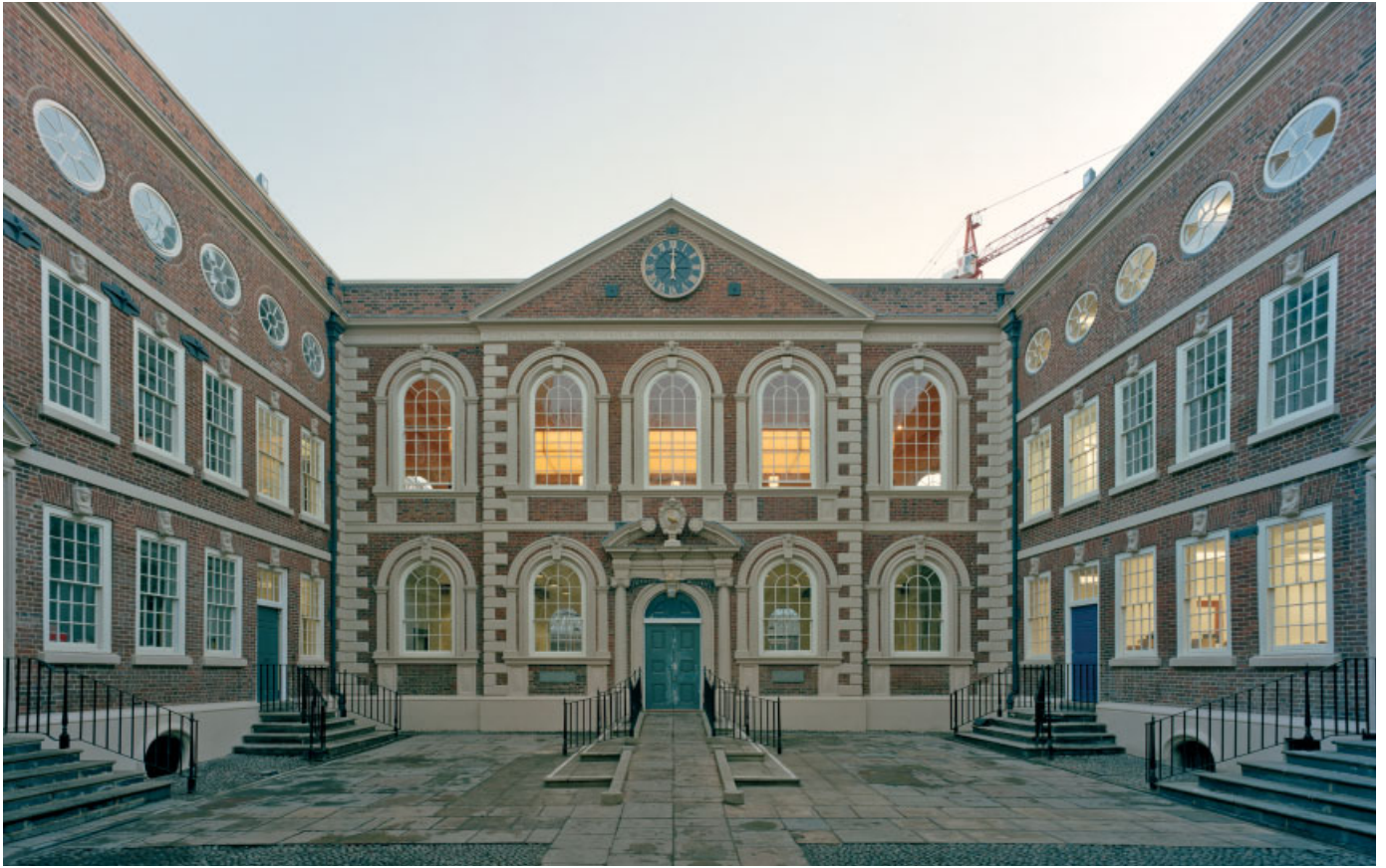
The principal entrance to the Bluecoat. The wing on the left suffered Second World War bomb damage, and the floorplates within are of 1950s concrete.
