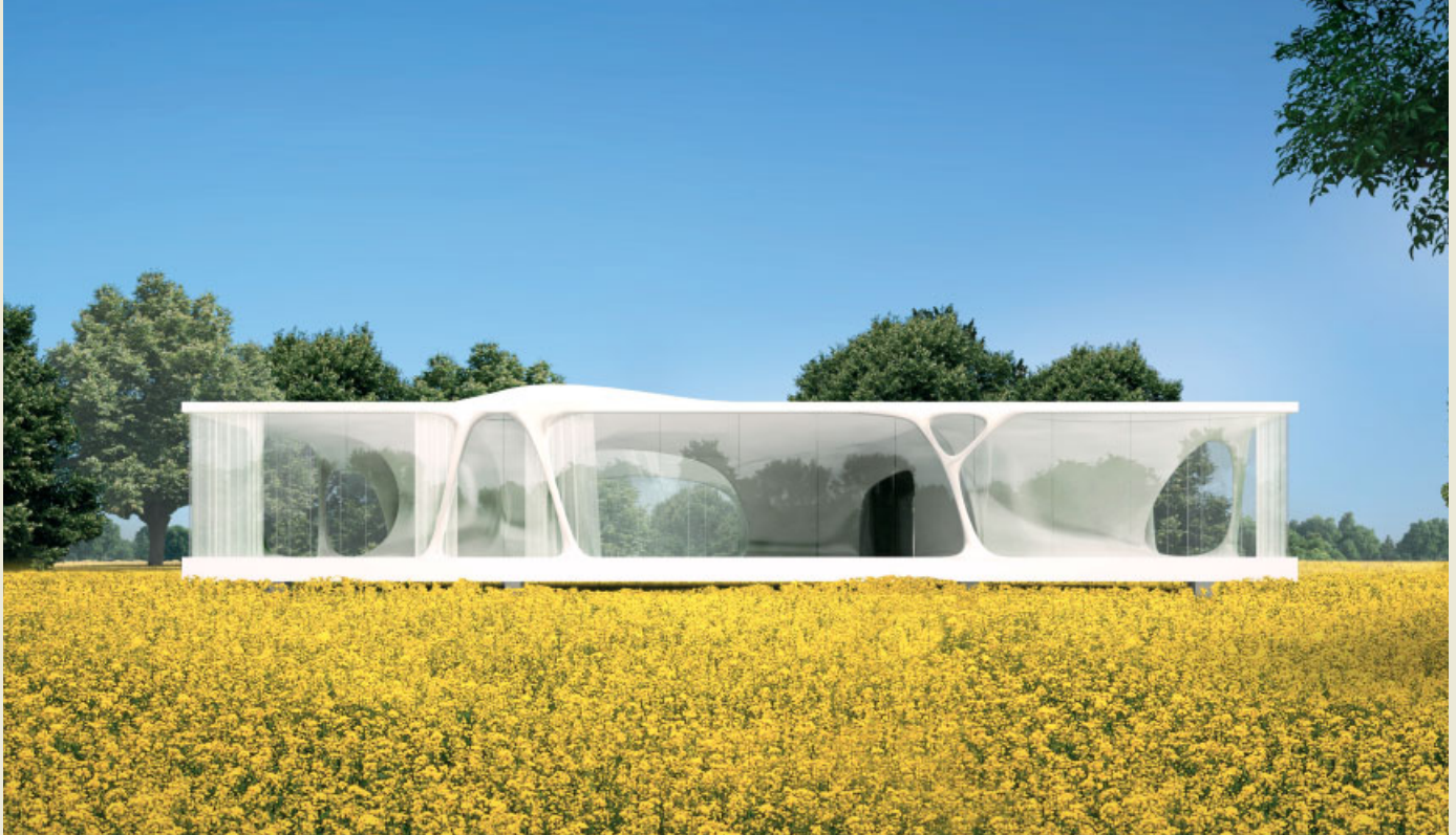
MAD's design for a low-energy, lightweight prefabricated house-pavilion to be made in China and shipped to Denmark for assembly.
